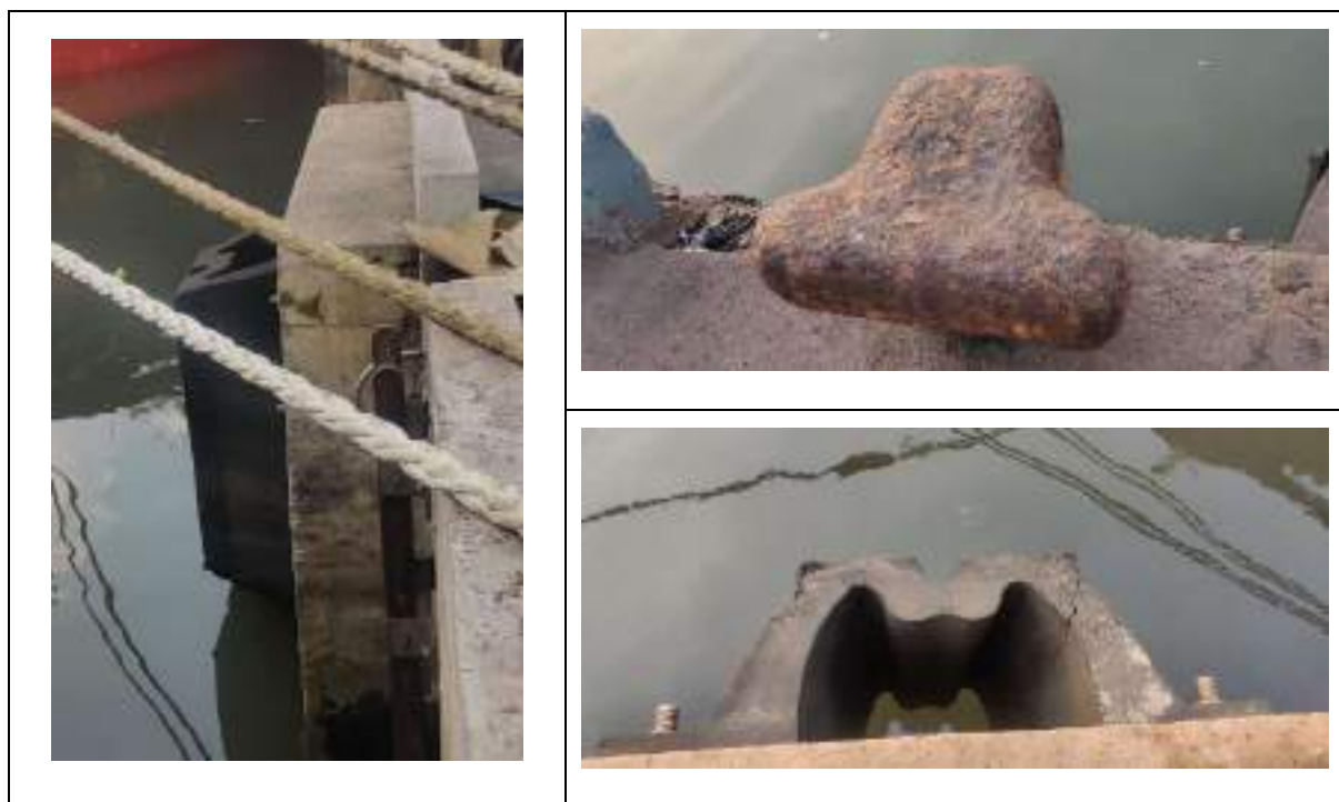
Figure 5-1 : Fenders and Bollards at EQ-06
