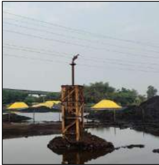
Figure 5-7 : Sprinkler type Dust Suppression System
